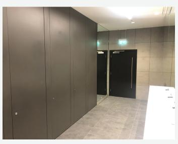
Our metal framed non-plumbed washroom panelling system, Frameduct, was specified for the WCs and urinals. The sturdy metal-framed panelling system makes for quick installation while the 90° linear bearing hinged panels offer easy ongoing maintenance. Further elevating the look of the washrooms, a bespoke herringbone design was routered into the panels.
